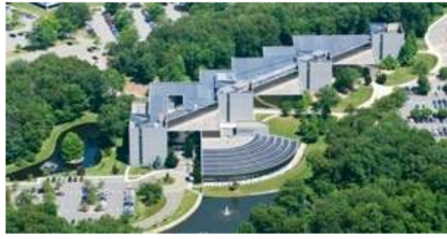
56 Roseland (Courtesy Mountain Development Corp.)
